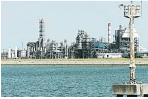
Space seeker: Other than oil refineries, Jurong Island (above) will also be home to the Jurong Rock Cavern; 'Besides using the surface as a resource to build on, we are trying to use the underground as an additional resource,' says Mr Ong (next photo)
